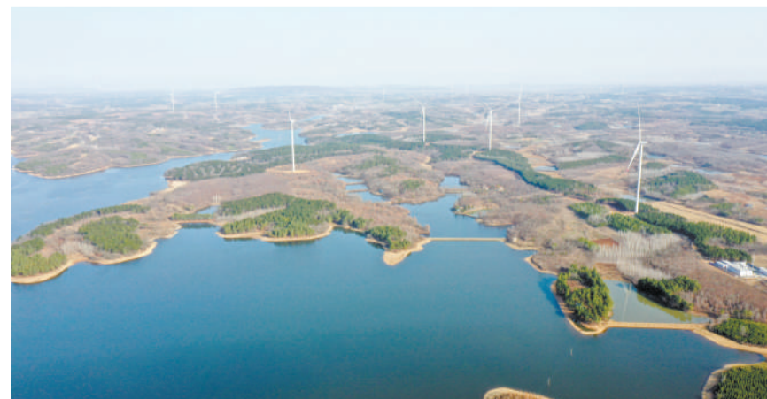
With a total installed capacity of 47.5 megawatts, the Zhuying and Zhangpuying wind power plants in Chuzhou, Anhui province, were officially connected to the grid on Dec. 19. (PHOTO: XINHUA)
