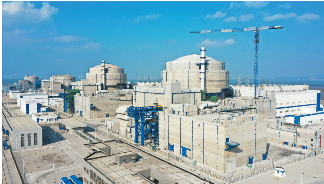
Fuel loading has started at China's second nuclear power unit using Hualong One technology, after the first one entered commercial operations earlier this year. (PHOTO: XINHUA)
