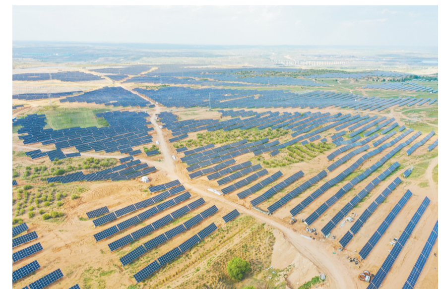
An aerial view of the solar photovoltaic power station at the mining subsidence area in Wulanmulun town, Ordos city. (PHOTO: XINHUA)
