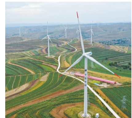
A wind power plant in Dingxi, Gansu province. (PHOTO: XINHUA)
